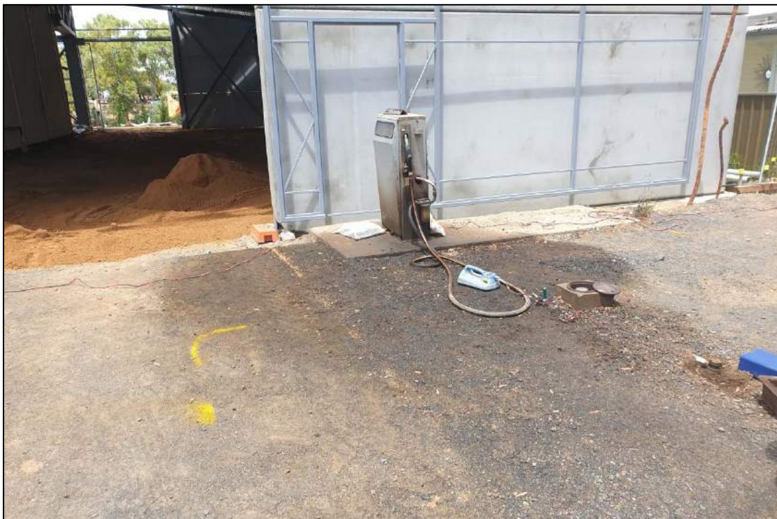
Photograph 9: Image of fuel pump with associate fill / dip points and approximate mark-up of tank footprint; hydrocarbon staining apparent on soil surface, facing south (8 December 2020). Location BH123 situated near inferred location of UST
